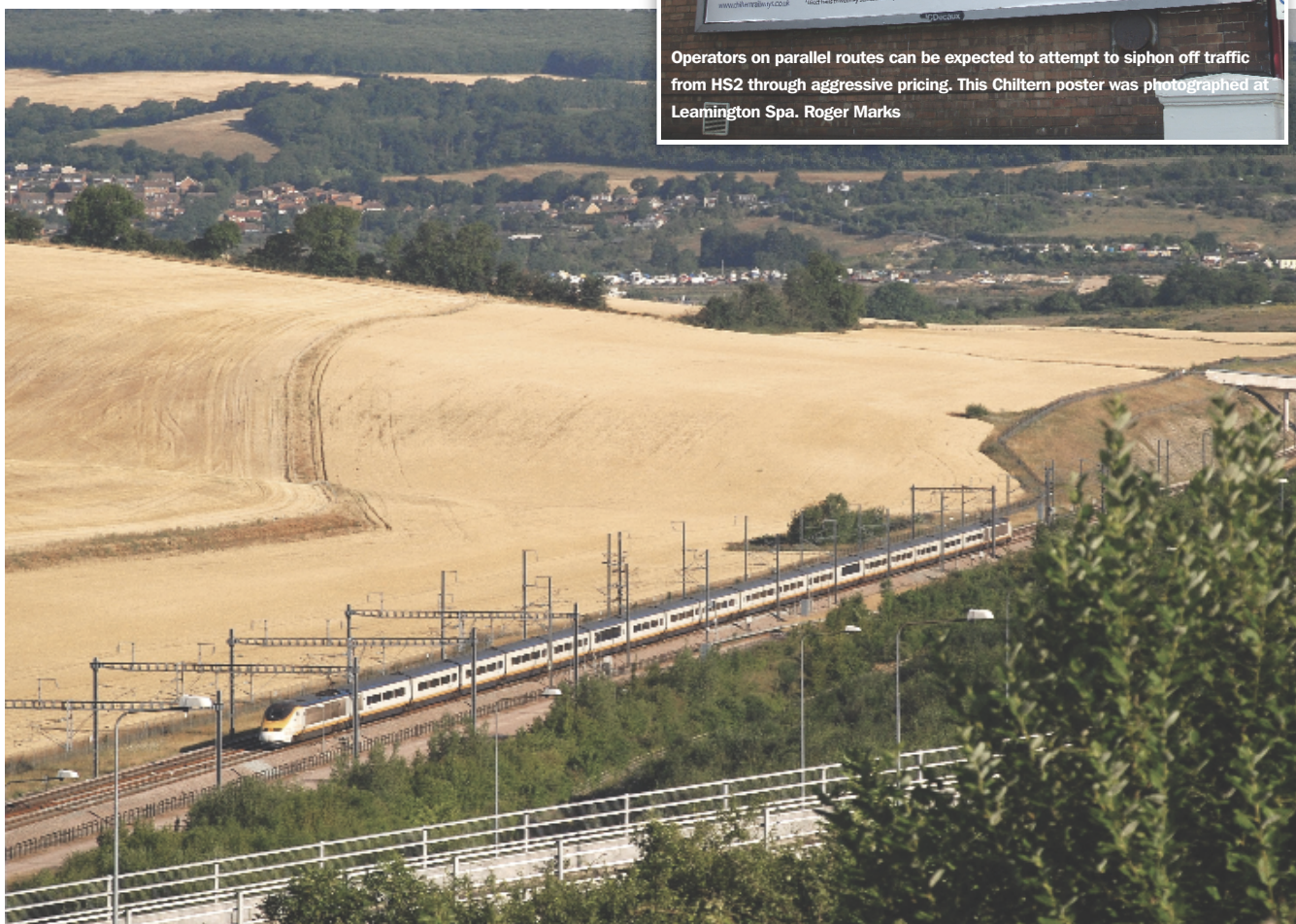
The 07.27 St Pancras International - Paris service powers up the Nashenden valley towards the North Downs tunnel on HS1 on 28 July 2010. David Staines
