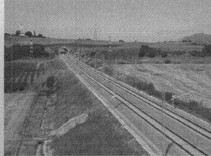
Example of railway on embankment Rome - Naples
