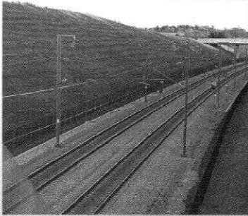
Example of railway in cutting High Speed 1
