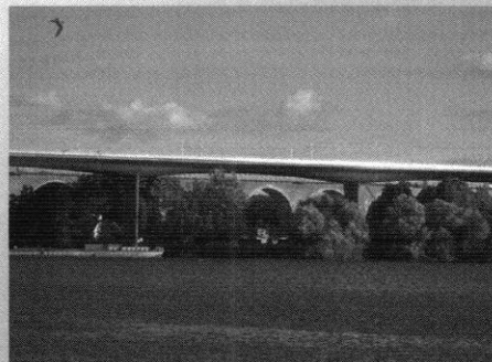
Arsta viaduct (Arup)
