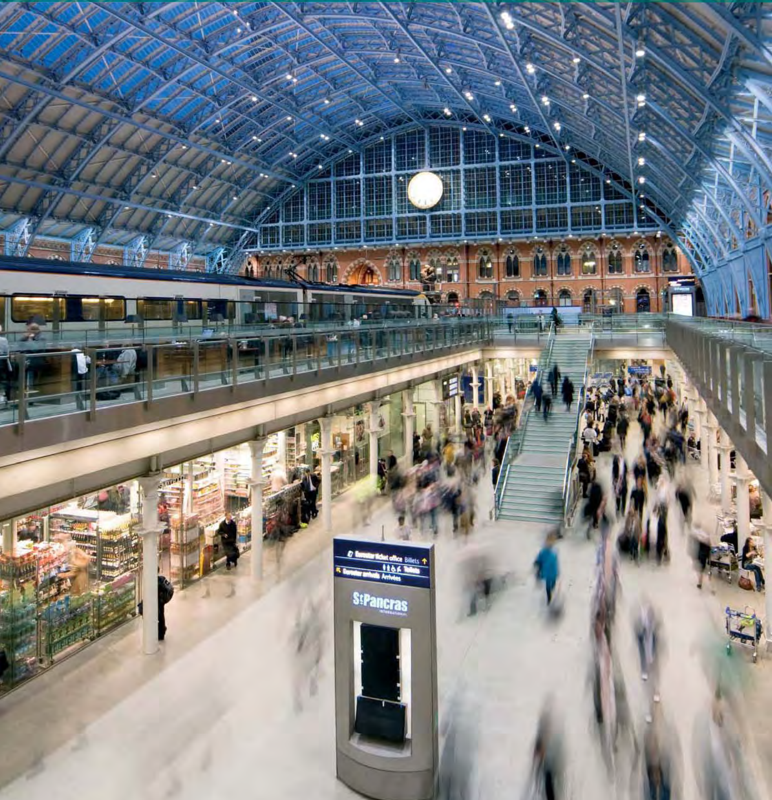
St Pancras Station, restored, expanded and reopened in 2007 as the terminus for High Speed One.
